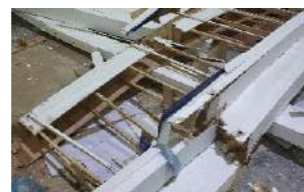
Construction Templates & Waste Wood
